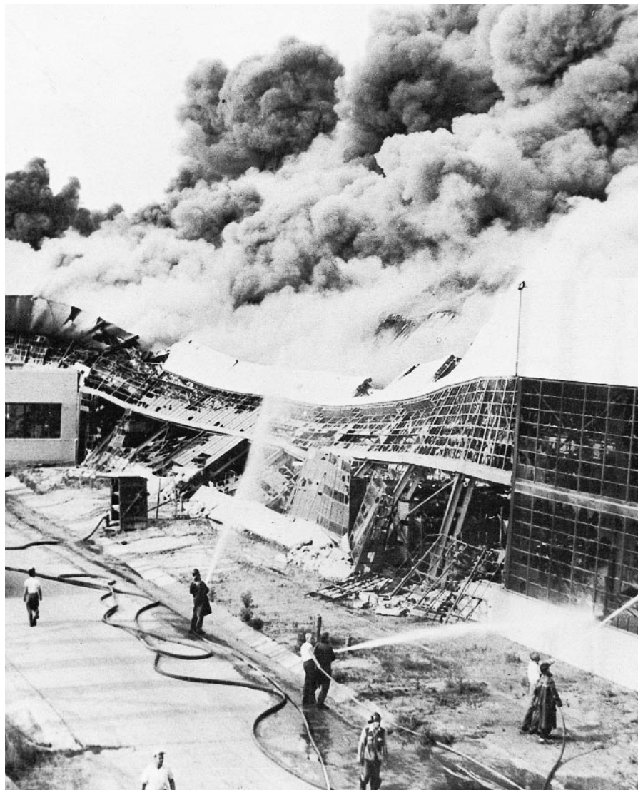
General Motors plant in Livonia, Michigan was unprotected metal construction (see text).
