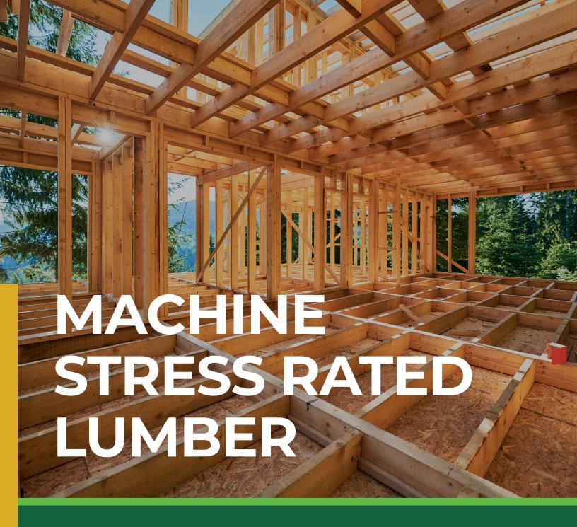
Available in various lengths, strengths, and stiffness ratings, our **Hem-fir MSR** product provides predictable performance for demanding engineering design criteria such as roof trusses and beams.
